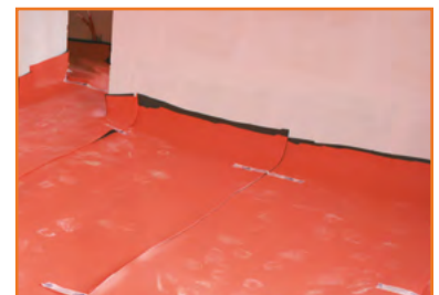
Rise the underlay alongside the wall ( \pm 15 cm)
