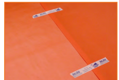
Keep the overlap maintained with the adhesive provided
