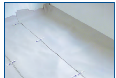
Rise the underlay alongside the wall (±15 cm)
