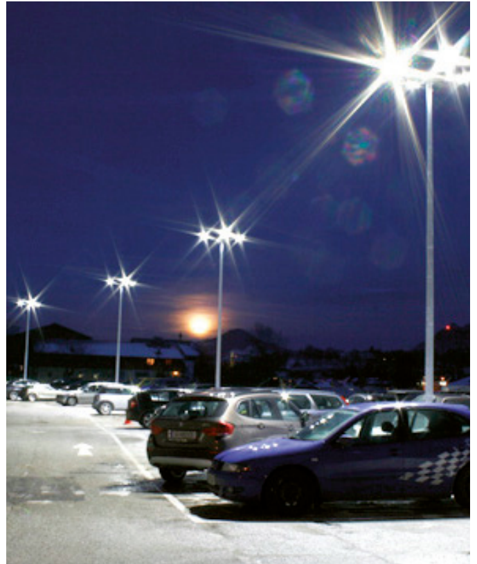
EDP No. 91124, car park, Park and Ride
