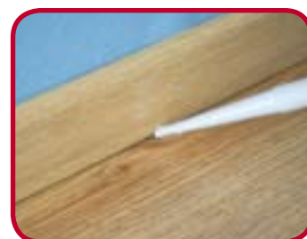
5. Attach the skirting board a few millimetres above the parquet flooring, then fill the gap with sealant
