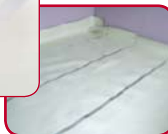
2. Apply the aluminium tape to the joints
