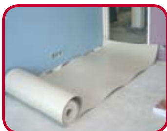
1. Unroll InsulSound wall to wall, leaving a surplus running up each wall
