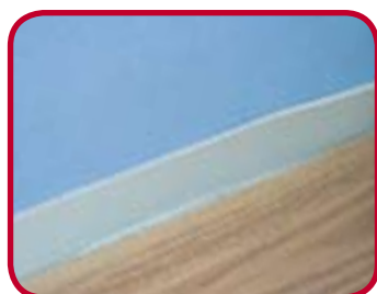
3. Place the parquet flooring, leaving the surplus underlay
